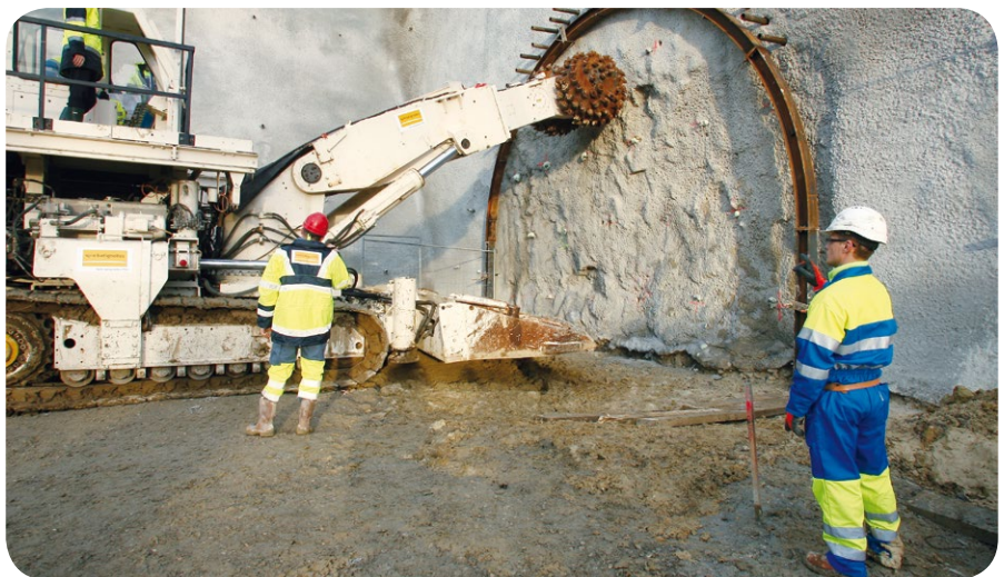
➔ Boring the 574-metre long tunnel
